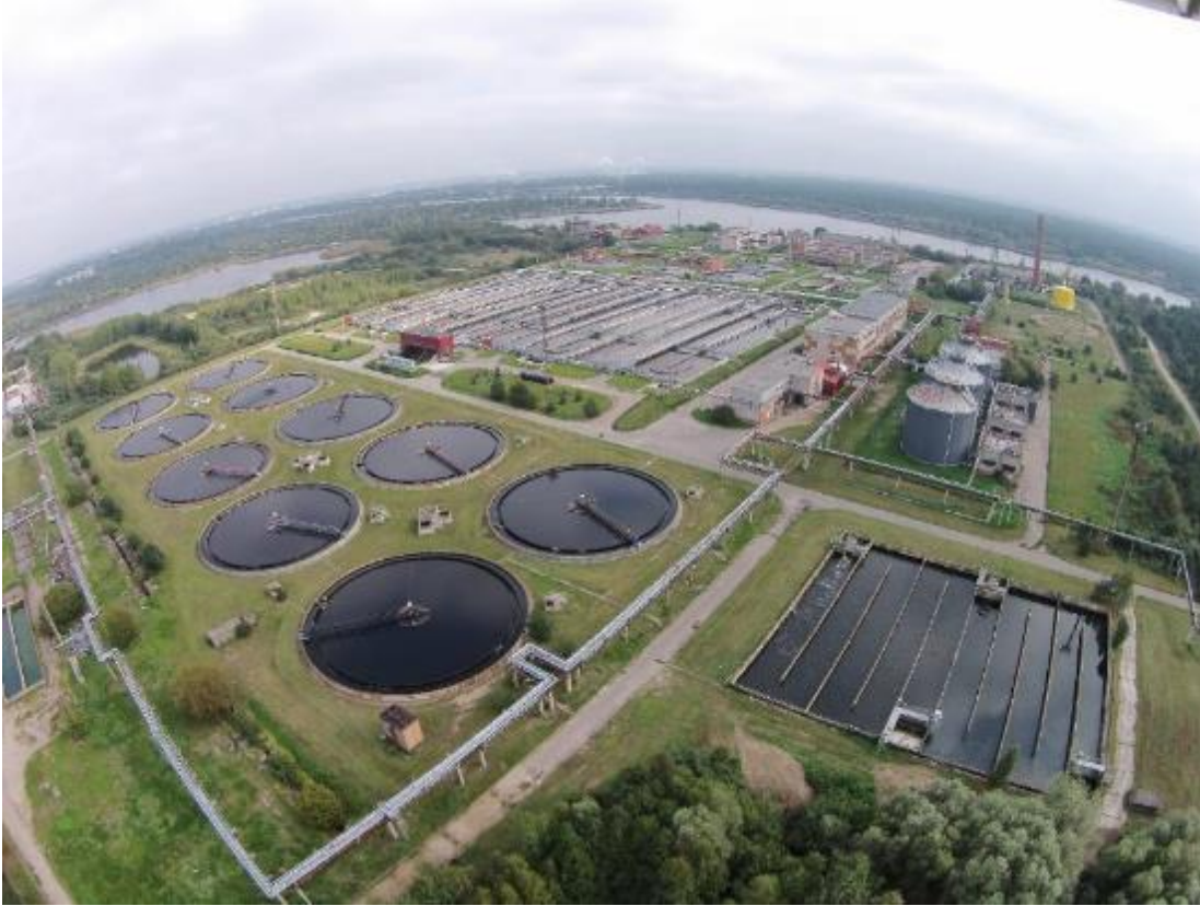
Figure 1.2. Daugavgrīva biological wastewater treatment plant (photo “Rīgas ūdens”).
